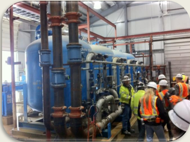
LMPT touring Kensington Water Treatment Facility
