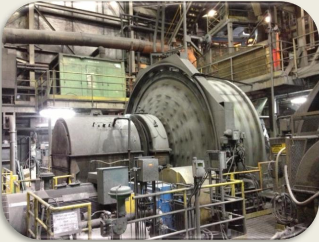
Greens Creek mill facility
