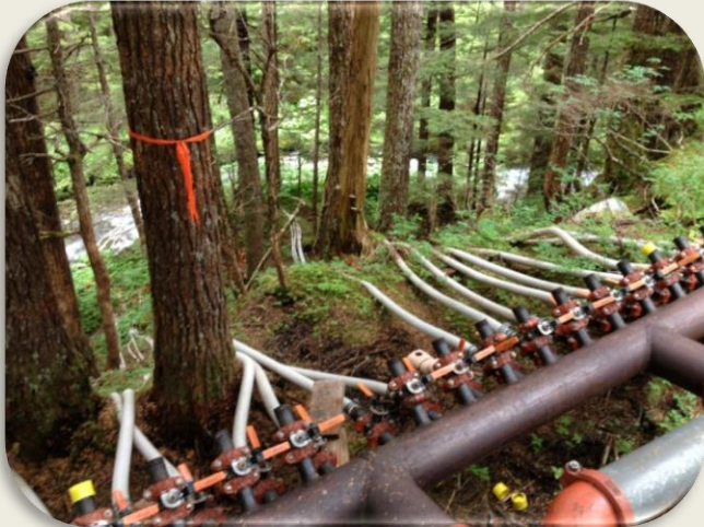
Kensington water discharge diffuser ("The Octopus")
