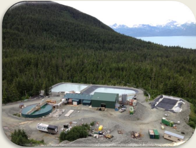
Kensington Water Treatment Facility
